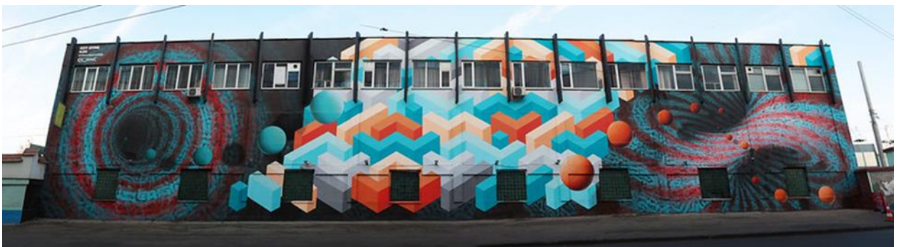
The building of the Chişinău Trolleybus Depot. Moldova, Chişinău, 146 Dosoftei str.
